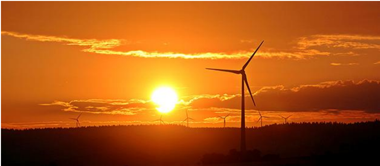
Fircroft, 2017. $110 MILLION BOOST FOR KAZAKHSTAN RENEWABLE ENERGY
