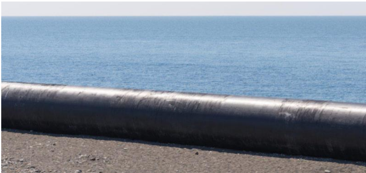
Euractiv, 2017. Central-Eastern European pipeline gets go-ahead
