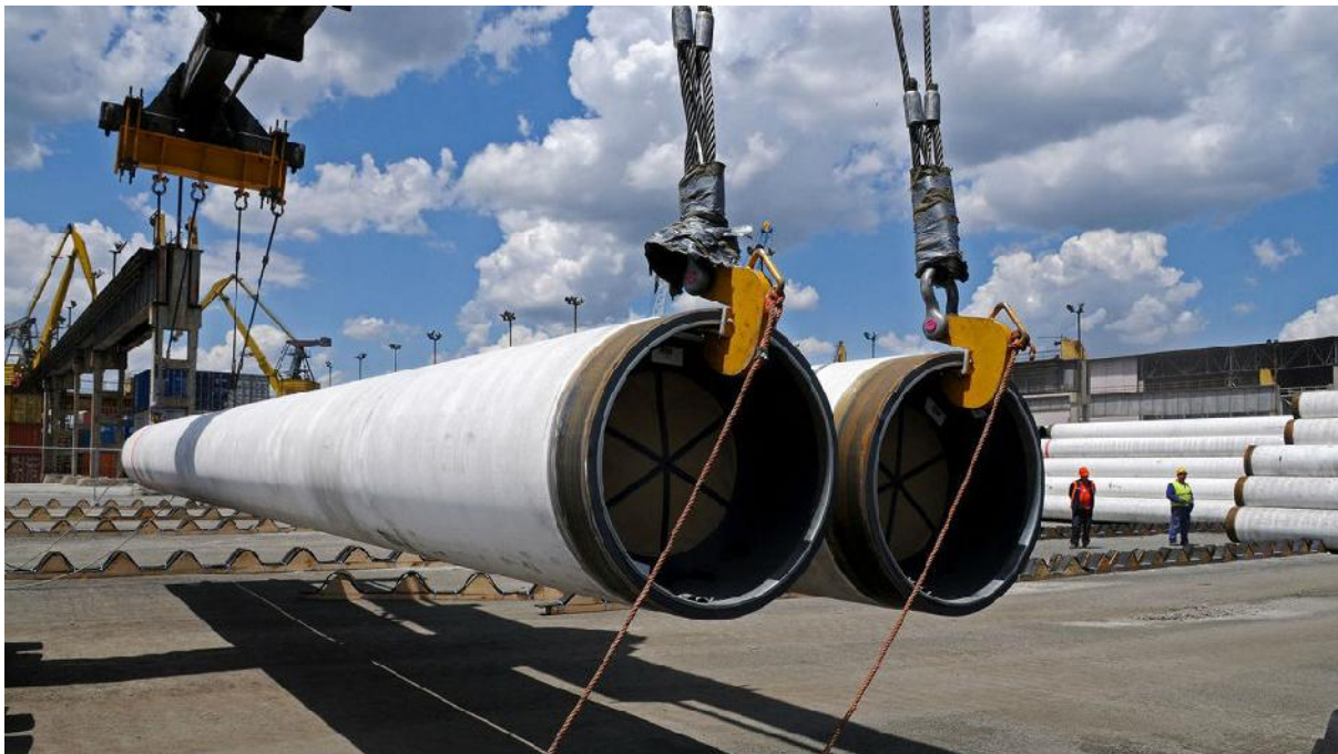
The Maritime Executive, 2017. Construction of TurkStream Offshore Pipeline Commences
